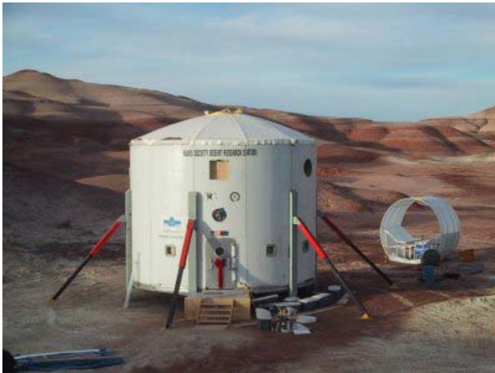
Figure 5 The MRDS under construction in SW Utah 9
